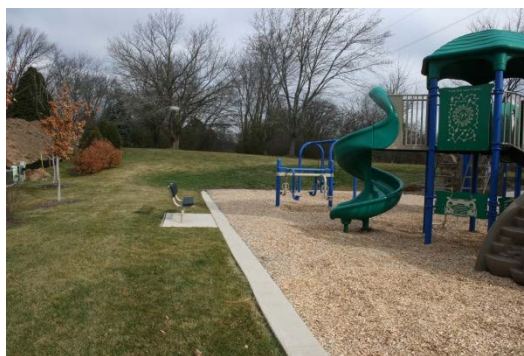
Concrete Edge Restraint and Bench Pad
